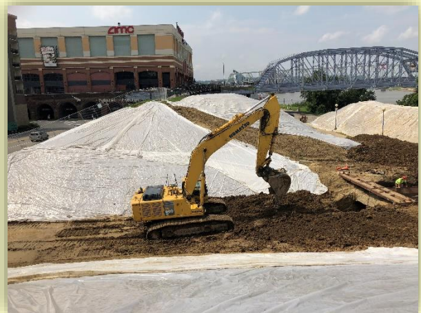
Aqua on the Levee Storm Sewer Project
